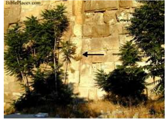
"Seam" on Eastern Wall
